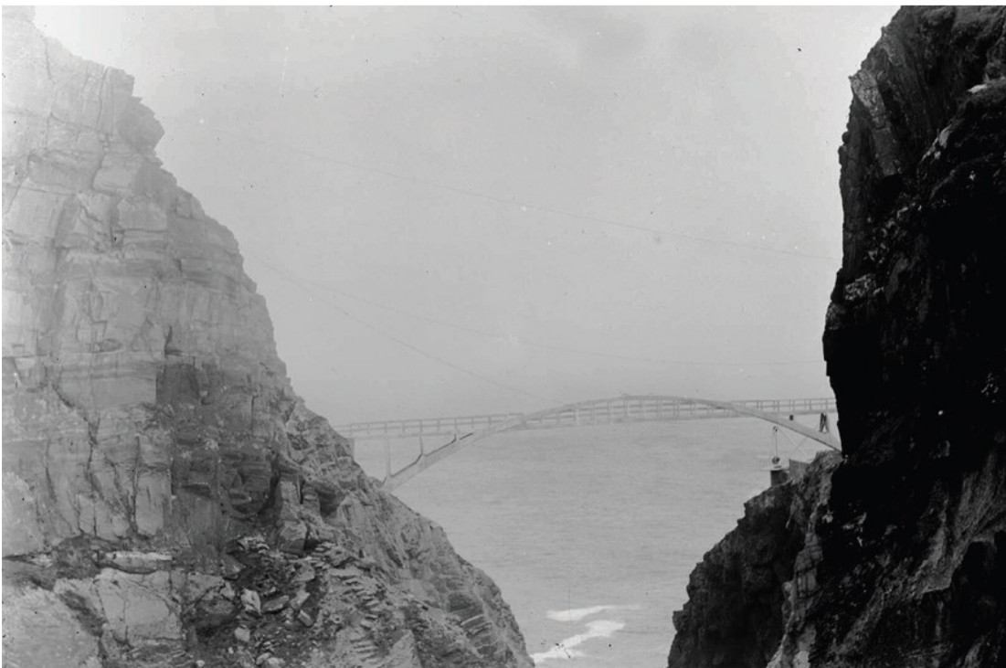
"Now when the bridge is erected the beauty of the design can be seen. At a distance it looks like a monster spider's web hanging in the air, its graceful curve of 30 feet adding much to its attractive appearance while its long span of 172 feet over the chasm and often times raging sea over 150 feet below seen against the bold precipitous bluffs of the Mizen Head side-view, leaves a picture in the mind's eye scarcely ever to be forgotten." – Florence McCarthy
