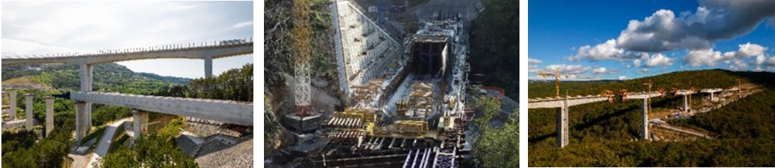
Figure 8: Three viaducts, three different construction methods
