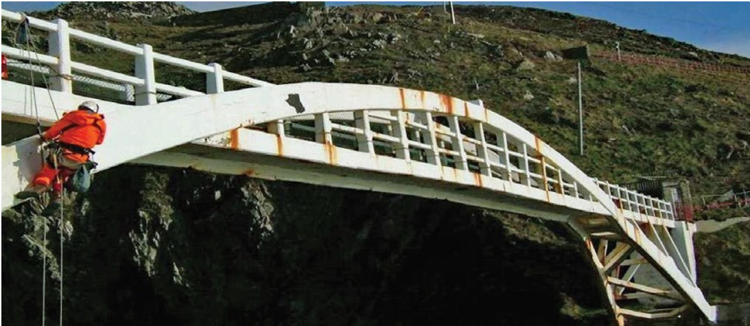
Specialist Abseil Engineers inspect the bridge (2004?).
