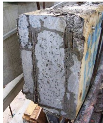
(Left) Ridley's arch rib design. (Middle) 3D depiction of an arch rib makeup. (Right) Sliced section of an arch rib (photo taken during demolition).
