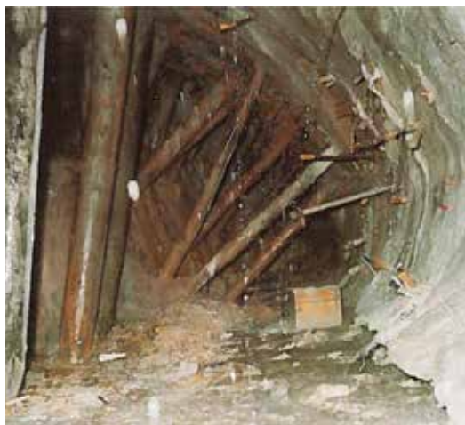
Slika 1: Razmere pri izkopu skozi prelomno cono v Werfenski formaciji [1] in shema uporabljenega podpornega tipa pri reprofilaciji. Conditions during excavation through the fault zone in the Werfen Formation [1] and the scheme of the support type used during reprofiling.
