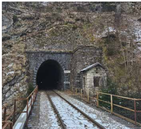
Slika 1: Pogled na severno (levo) in južno (desno) portalno konstrukcijo predora View of the northern (left) and southern (right) portal structure of the tunnel
