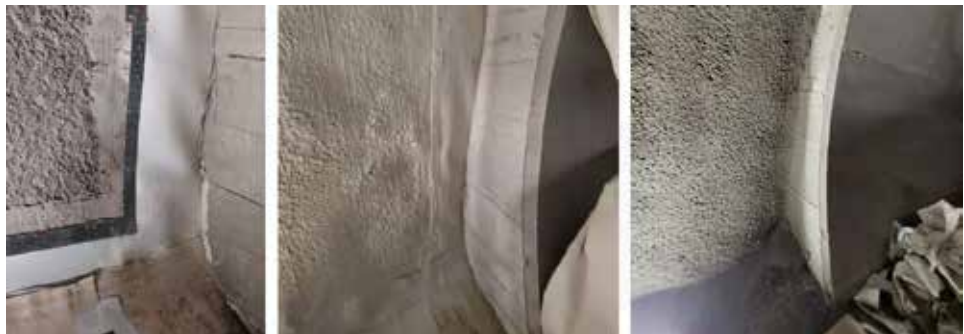
Fig. 9: from left to right: preparation of the overlapping onto TPO membrane; fresh MasterRoc MSL 345 applied onto TPO membrane; MasterRoc MSL 345 covered by secondary sprayed concrete lining
