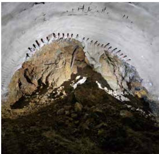
Slika 10: Izpadanje blokov dolomita v fazi izkopa kalote v coni nizkega nadkritja. / Block failure of dolomite during the excavation of the top heading in the low overburden zone.
