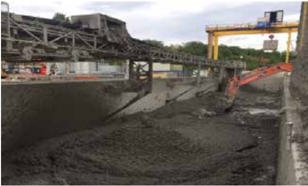
Fig. 2: Example of a temporary deposit of spoil material of an EPB construction site. [19]
