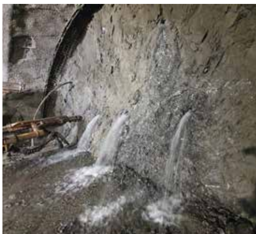
Slika 4: Dotok vode na območju Werfenske formacije z reprezentativnim podpornim tipom. Water inflow in the area of the Werfen Formation with a representative support type.
