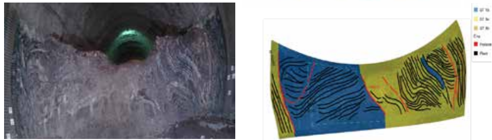
Fig. 9: Popis in fotografija izkopa stopnice na TM 2231,3 (17.11.2022). Description and photograph of the bench excavation at TM 2231,3 (17/11/2022)
