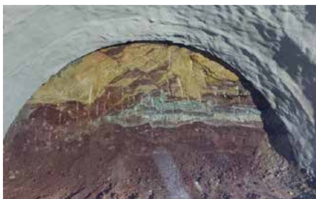
Slika 5: Primerjava izkopnih čel v rdečih in rumenih fino-zrnatih meljevcih in v tektonsko prettrtem dolomitu z vmesnimi plastmi peščenega meljevca. Comparison of excavation faces in red and yellow fine-grained marls and in tectonically fractured dolomite with interbedded layers of sandy marl.
