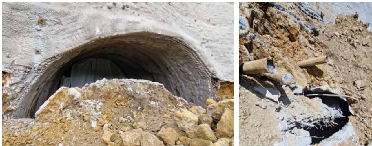
Slika 11: Preboj predora Konovo na južnem portalu z izvedbo ojačitve po robu preboja (levo) in detajlom preboja pod cevni ščit (desno). Breakthrough of the Konovo tunnel at the southern portal with reinforcement along the edge of the breakthrough (left) and a detail of the breakthrough under the pipe umbrella (right).
