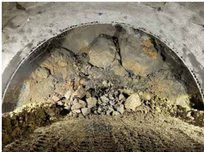
Slika 10: Izpadanje blokov dolomita v fazi izkopa kalote v coni nizkega nadkritja. / Block failure of dolomite during the excavation of the top heading in the low overburden zone.
