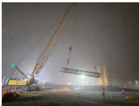
Slika 3: Vgrajevanje merilne opreme na armaturne koše diafragme, ki je potekala glede na dinamiko izvedbe del tudi ponoči. Installation of measurement equipment on the diaphragm reinforcement cages, which depending on the work progress was also carried out during the night.
