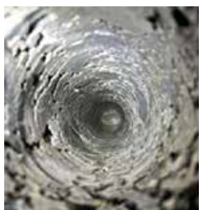
Slika 2: Oblogo sestavlja nearmiran beton, ki z globino preide v klesan blok apnenca The lining consists of unreinforced concrete, which with depth transitions into hewn limestone blocks.
