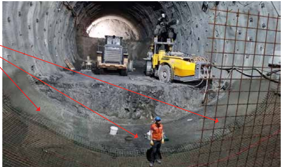
Fig. 4: Lokacija vgrajevanja mer-skih elementov v primarno oblogo talnega oboka v TM2506 in prikaz vgradnje merilcev specifičnih deformacij. Location of installation of measuring elements in the primary lining of the invert in TM2506 and installation of specific strain gauges.
