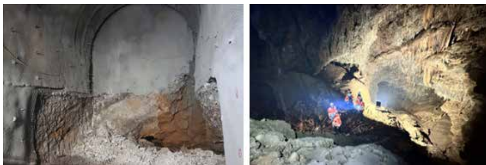
Fig. 5: Excavated tunnel face of deepening bench-invert in the service tube, at km 12+537 (left); the view from top heading in the main tube to the Entry chamber; the floor is filled with cave sediments and speleothems, stalactites are visible on the walls (courtesy of: M. Prelovšek).
