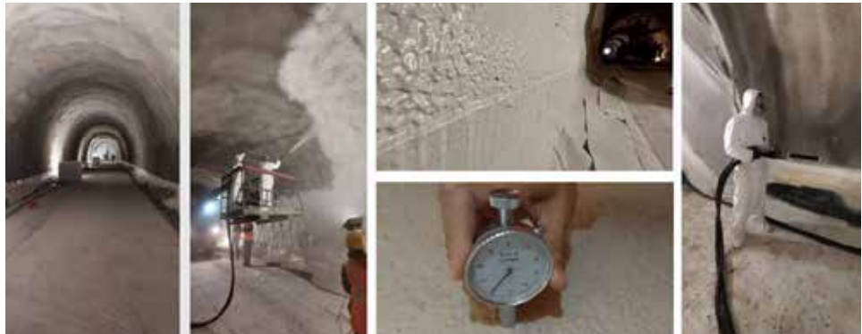
Fig. 8 from left to right: spraying of MasterRoc MSL 345; membrane freshly applied and measuring the Shore A; covering the membrane with sprayed concrete
