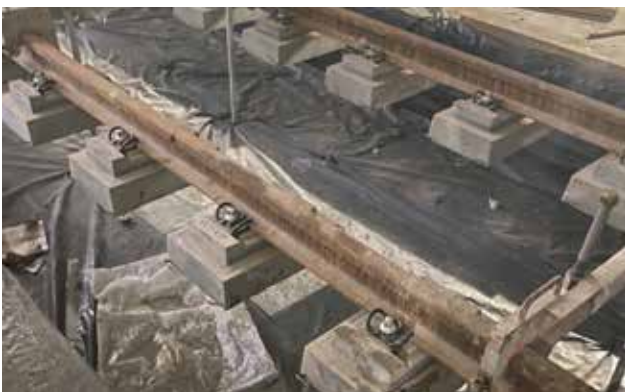
Fig. 3: Warsaw Metro original reinforcement and BarChip solution
