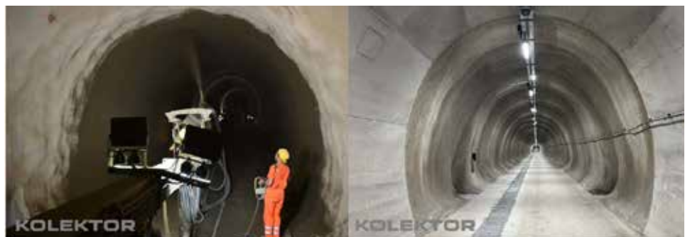
Fig. 10 from left to right: application of secondary lining of sprayed concrete onto the MasterRoc MSL 345; escape tunnel completed (CSL in contact with DSL)
