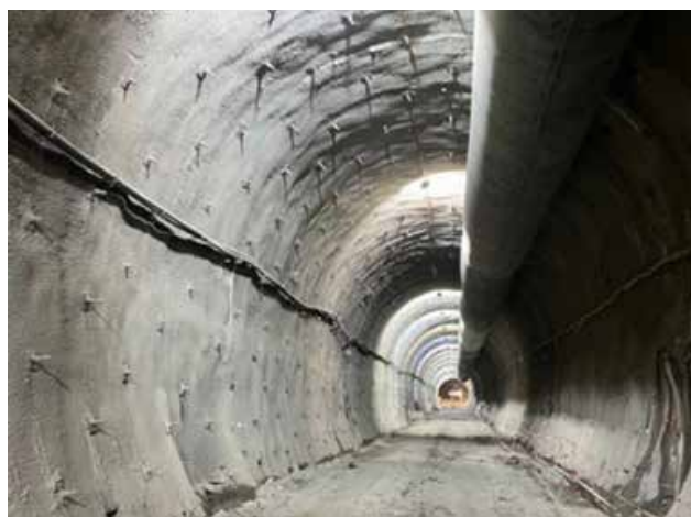
Fig. 4: Shotcrete lining under construction and ready lining with BarChip 54 and BarChip R65 fibre
