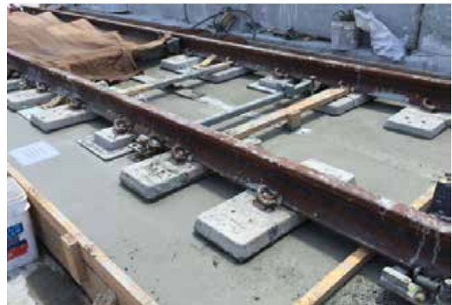
Fig. 1: Forrestfield Airport Rail Link, Perth, Australia and East Side Access, New York, USA
