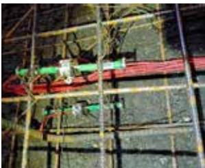
Fig. 4: Lokacija vgrajevanja mer-skih elementov v primarno oblogo talnega oboka v TM2506 in prikaz vgradnje merilcev specifičnih deformacij. Location of installation of measuring elements in the primary lining of the invert in TM2506 and installation of specific strain gauges.
